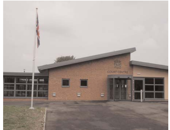
The new, video-equipped Bulford Military Court Centre
